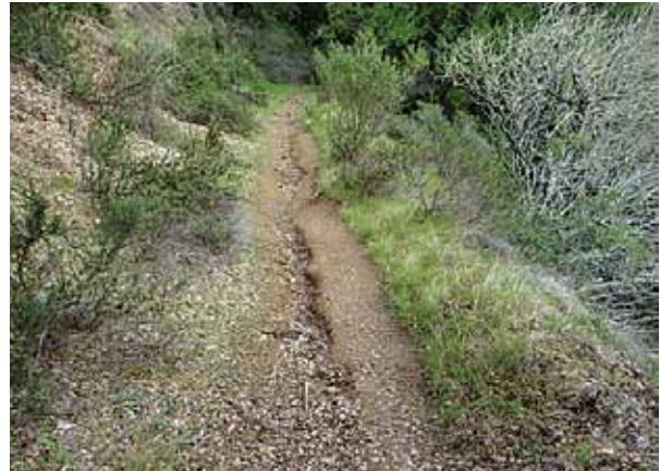
Figure 3.15 Shallow gulying is evident along this wide trail. The lack of cross drains results in runoff being concentrated, resulting in the observed erosion.
