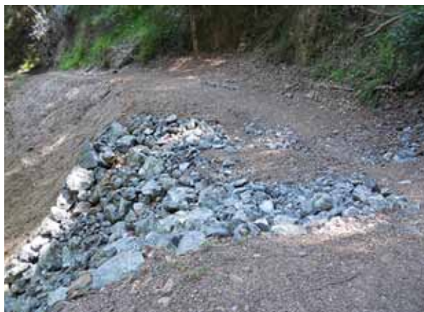
Figure 3.42 Rock ford on road-width trail.
