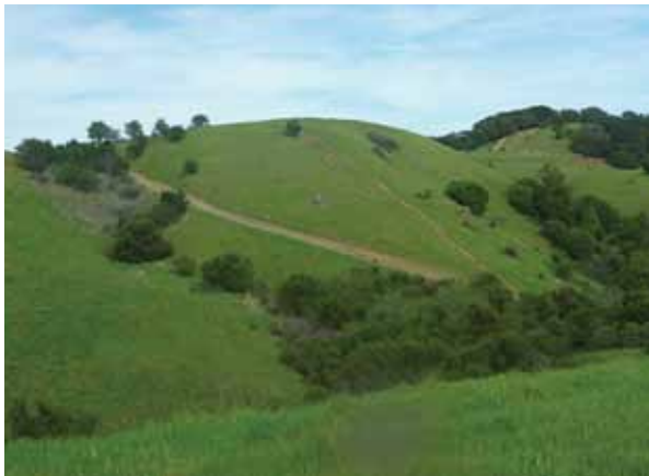
Figure 3.5 Steep road and fall line trail. Both are difficult to drain and experience much greater erosional problems compared to lower gradient trails.
