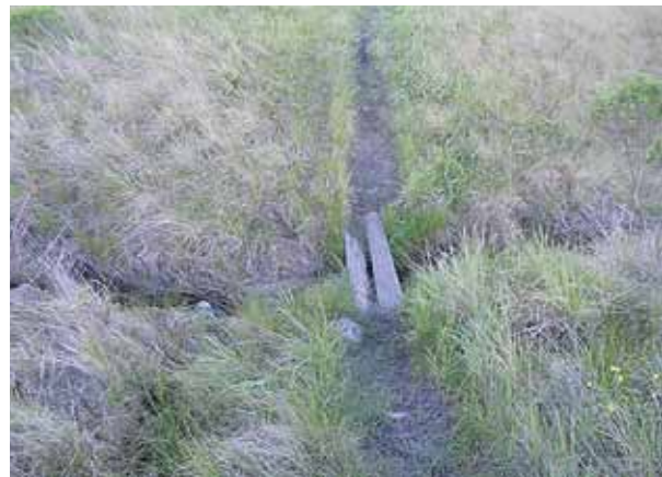
Figure 3.38 Informal puncheon over a small ephemeral watercourse.
