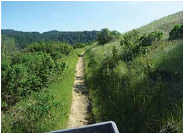
Figure 3.16 A narrow trail without drainage dips. The lack of dips and compaction of the tread has caused the trail to become entrenched.
