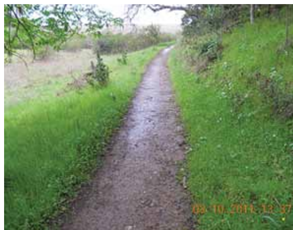
Figure 3.1 An example of good tread condition.
