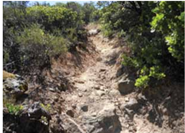
Figure 3.17 A deeply entrenched and poorly drained trail. Treatment of this trail will be difficult due to the steep grade and extensive entrenchment.
