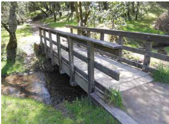
Figure 3.37 Functional wood foot bridge.
