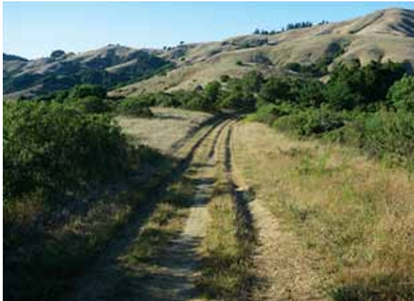
Figure 3.2 An example of fair tread condition.
