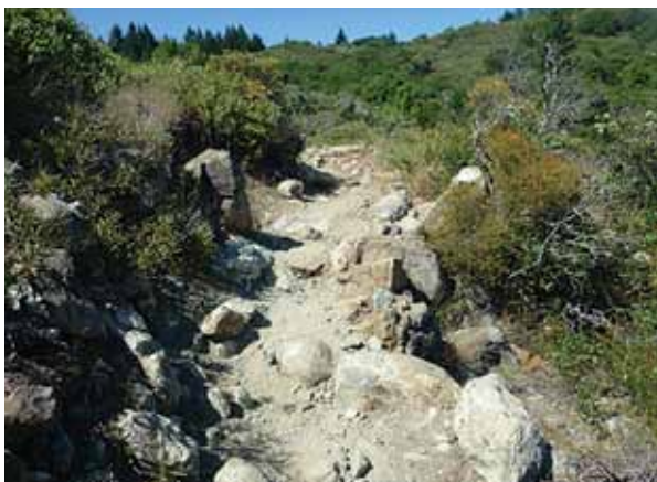
Figure 3.23 Highly irregular tread surface with continuous obstacles. This narrow trail is routed through serpentinite bedrock.
