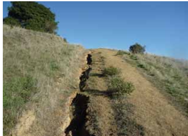
Figure 3.6 Erosion along steep (>15% grade) trail segment.
