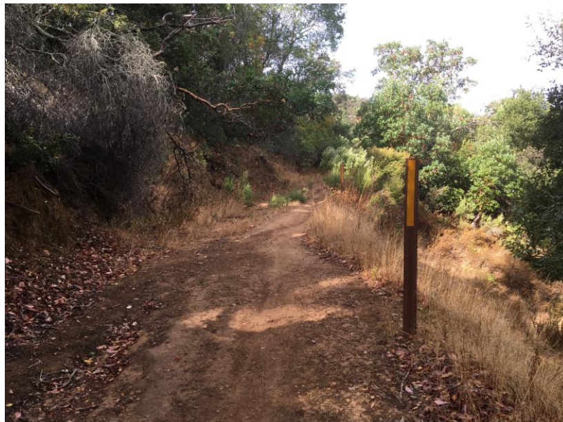
Photo 5: Ponti Fire Road (Landslide site)
