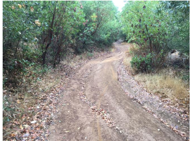
Photo 4: Rutting in Ponti Fire Road
