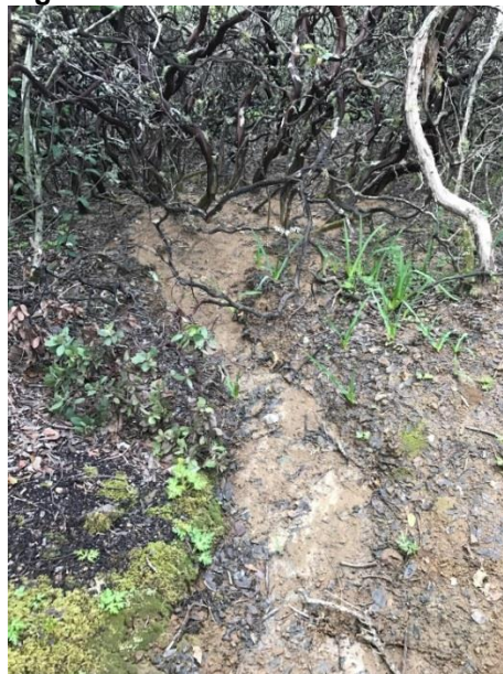
Figure 11: Erosion from Trail
