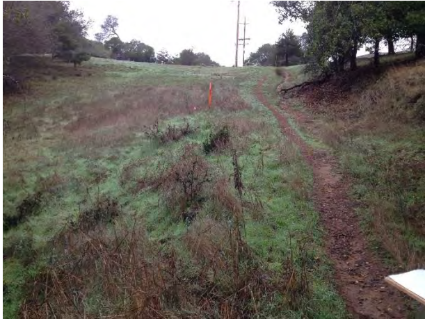
E – upper portion of existing trail. Grade could be reduced by realigning so as to traverse the area at left
