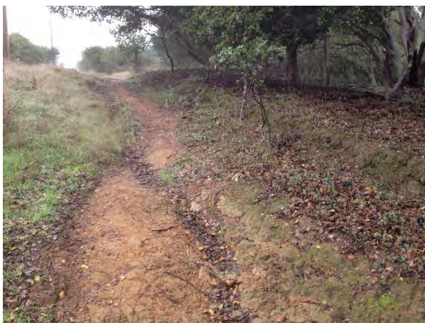
C – the same vicinity as (B), looking uphill. Note exposed weathered rock.
