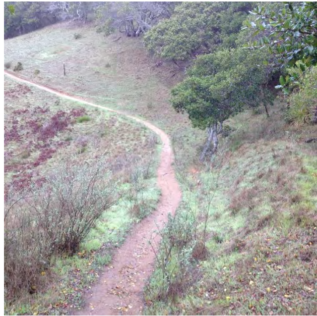
J - segment has approximately 20% slope, but good sight distance, and interval is short
