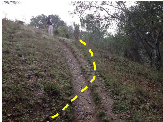
D – this steep segment (22%) could be reduced by realignment (realignment 1 on Figure 20)
