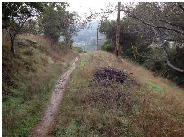
D – upslope portion of trail, looking downhill. The trail could be routed around the pole at right to reduce overall grade in this segment
