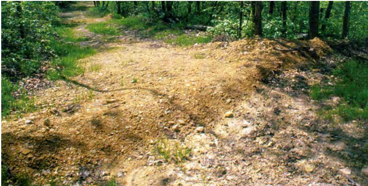
Example of a water bar drainage diversion (photo – Cornell University)
