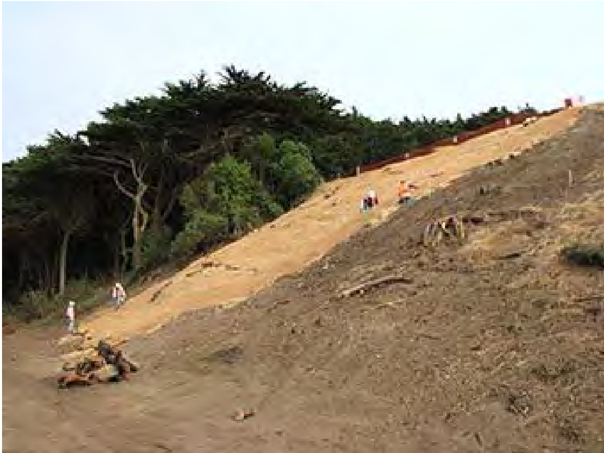
Example of erosion control mat being placed (photo – Go Native Restoration)
