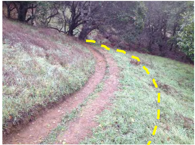
H - the slope in distance is steep; could be reduced by realignment 2
