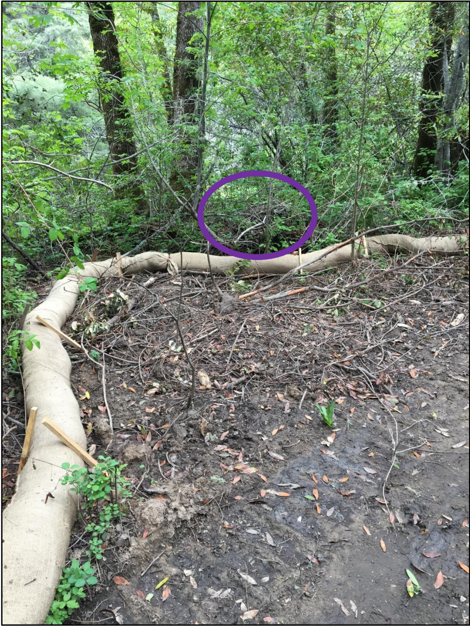
Attachment 3 – Photo of Geotechnical Investigation Site
