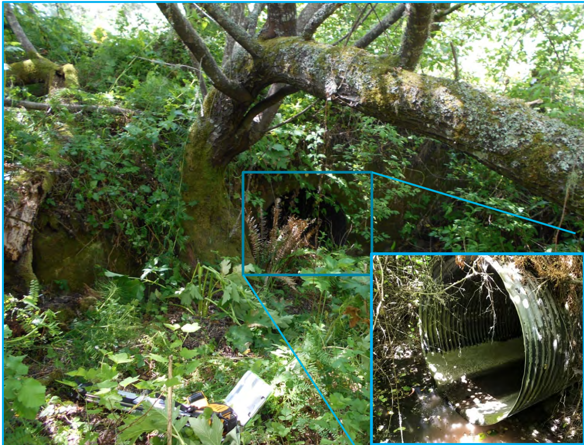
Figure 16. View Looking Downstream at the Culvert Inlet and Headwall on Lewis Gulch Creek at SR 1
