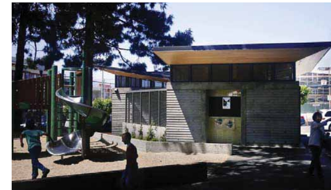
2 Restrooms + Event Service Facility
