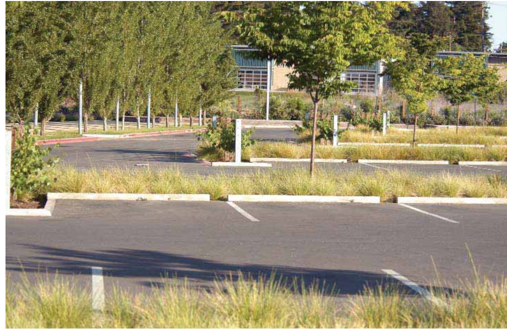
2 Vegetated Stormwater Treatment
